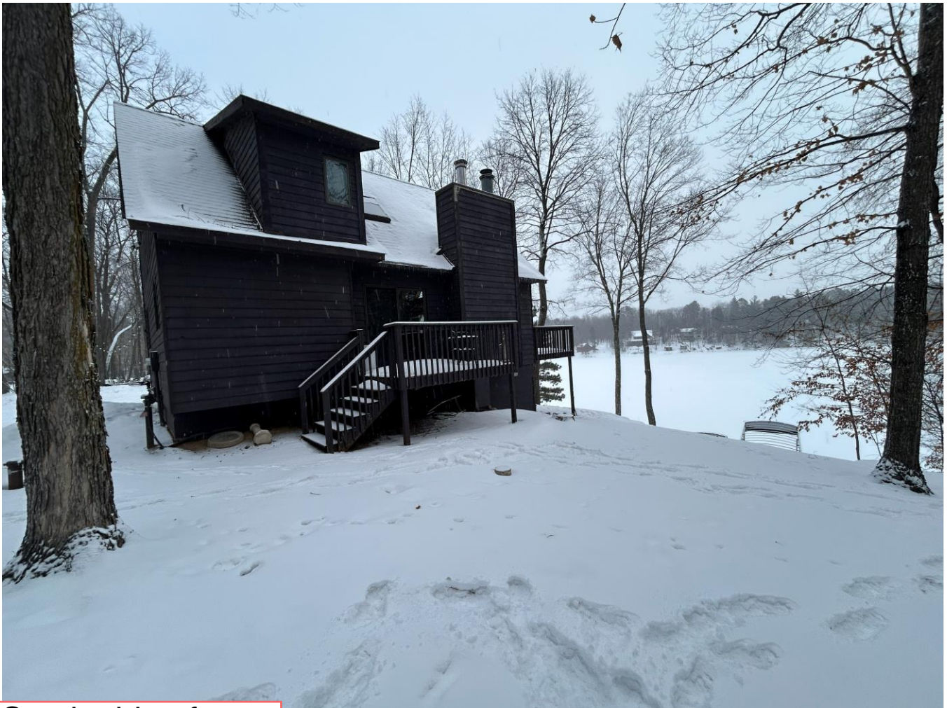
South side of house, facing north
