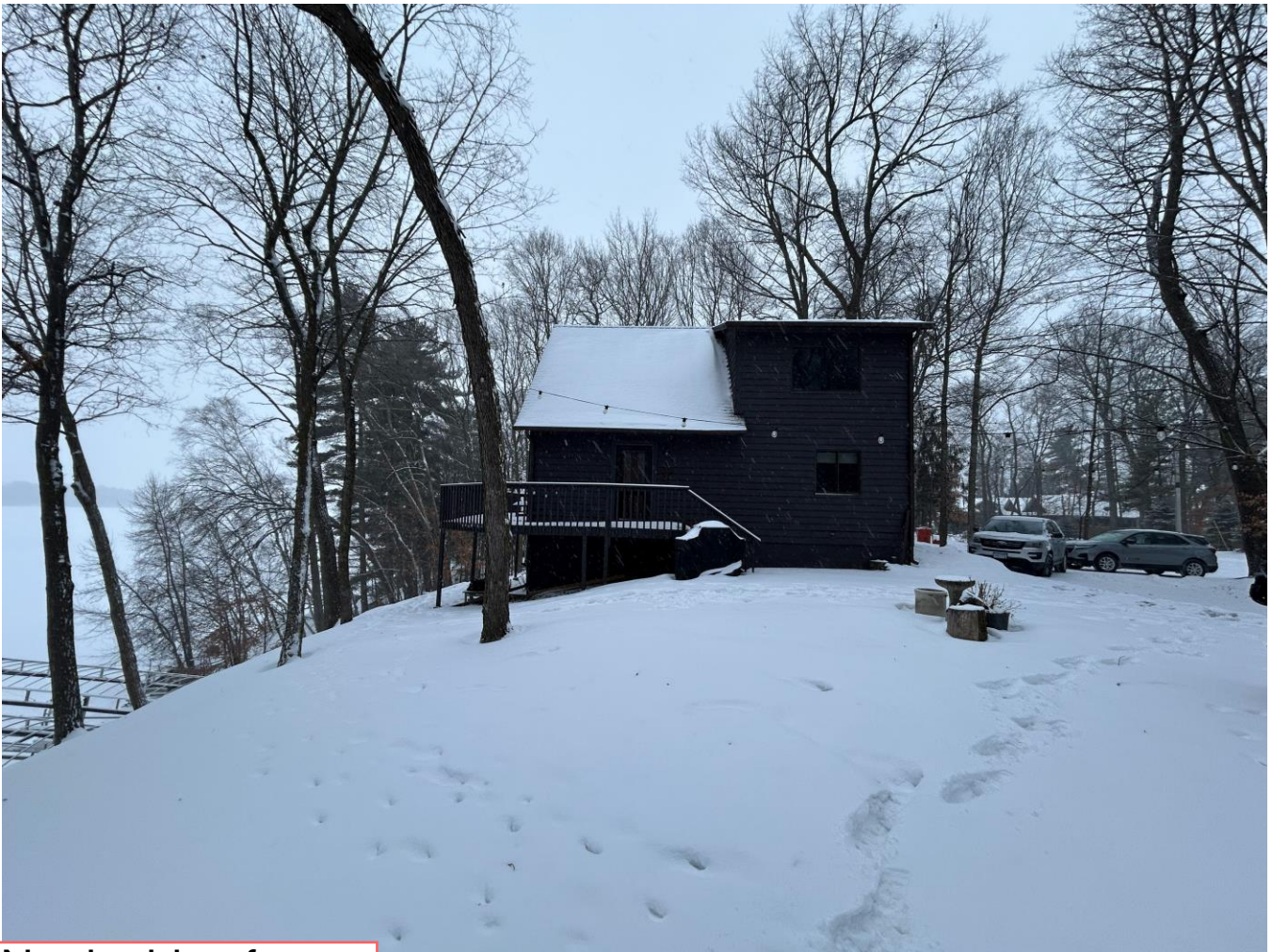
North side of house, facing south
