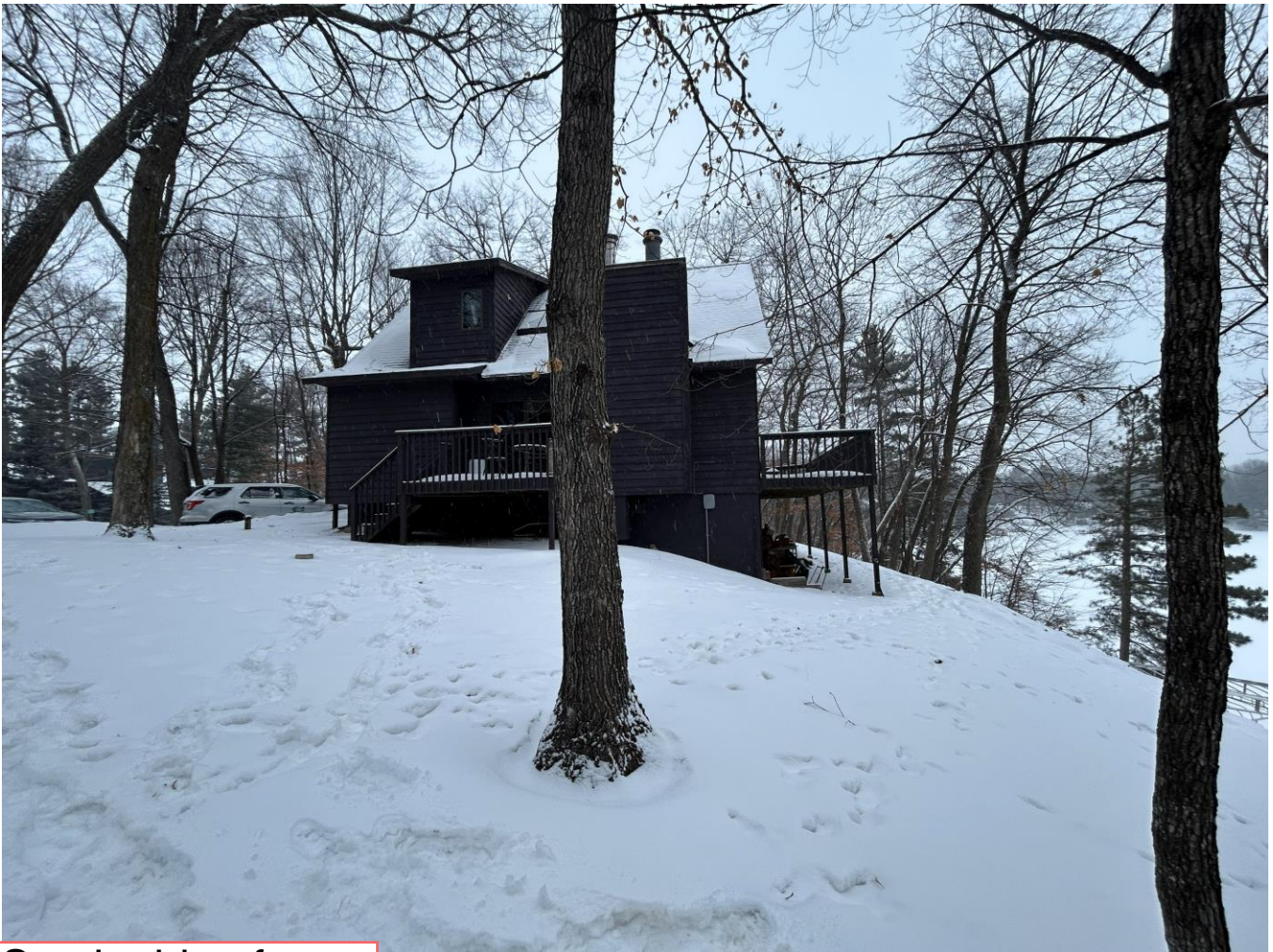
South side of house, facing north
