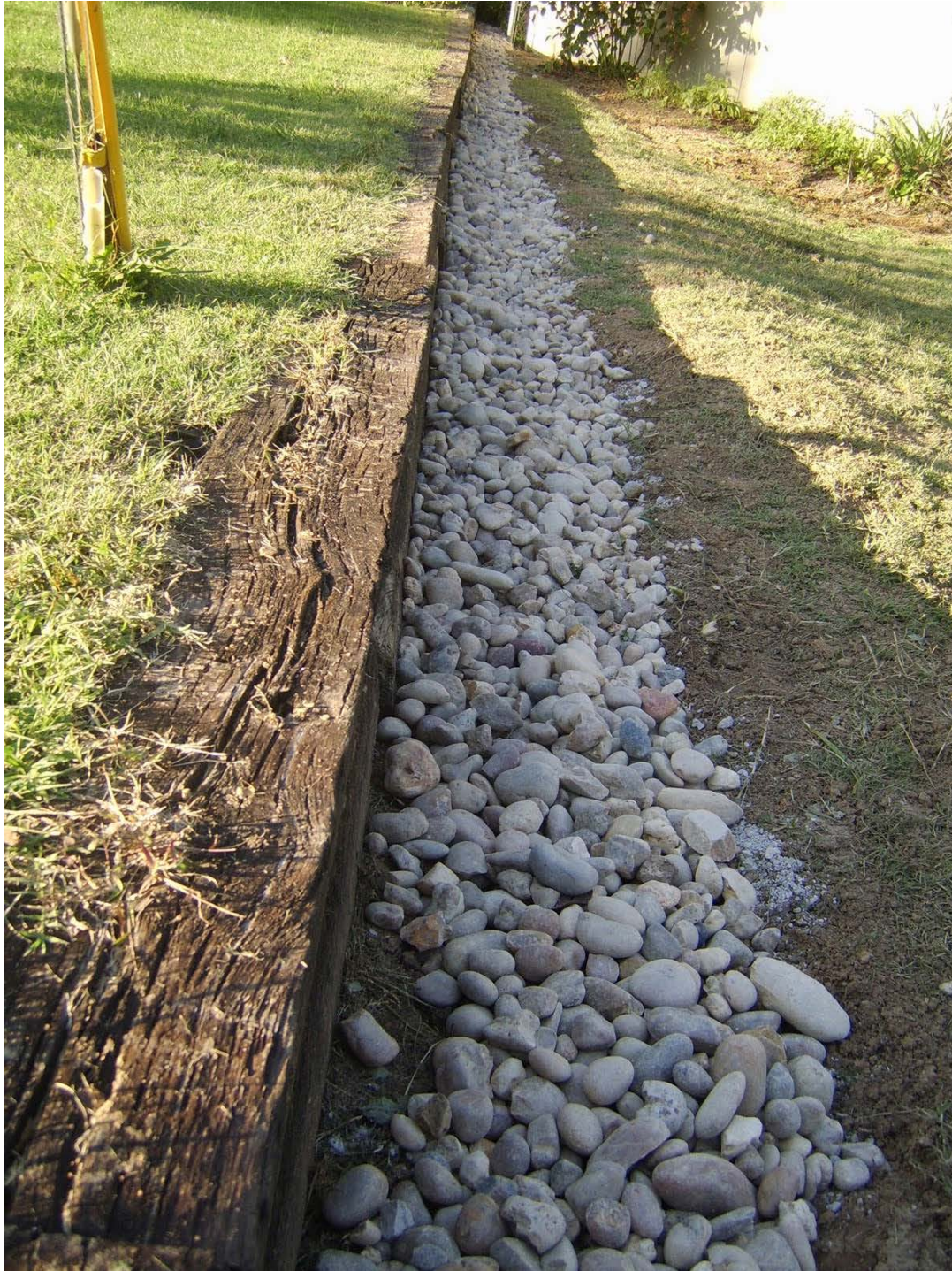
French Drain To Surface: along boulder wall
