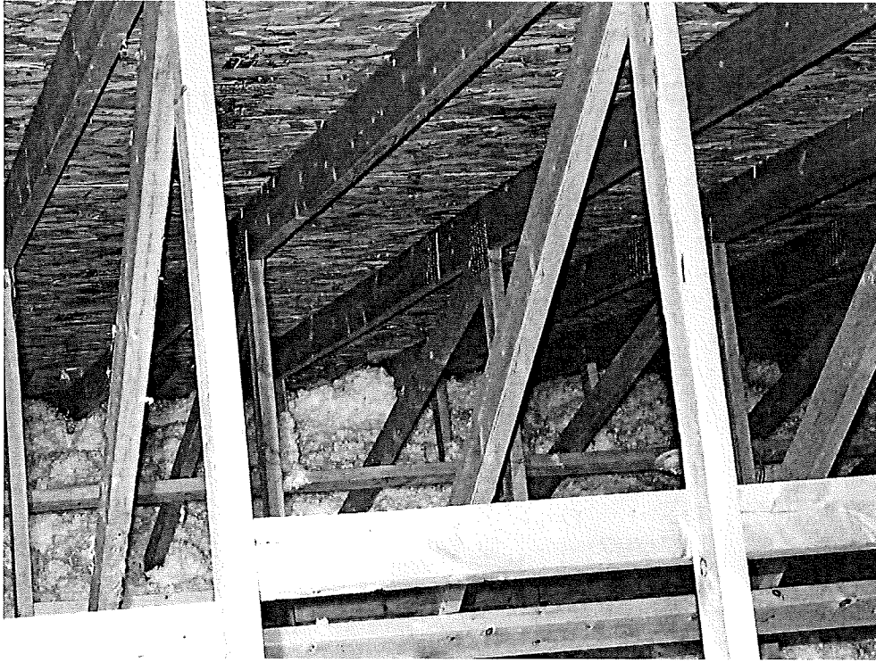
Photograph 13: Partial Air Chute
