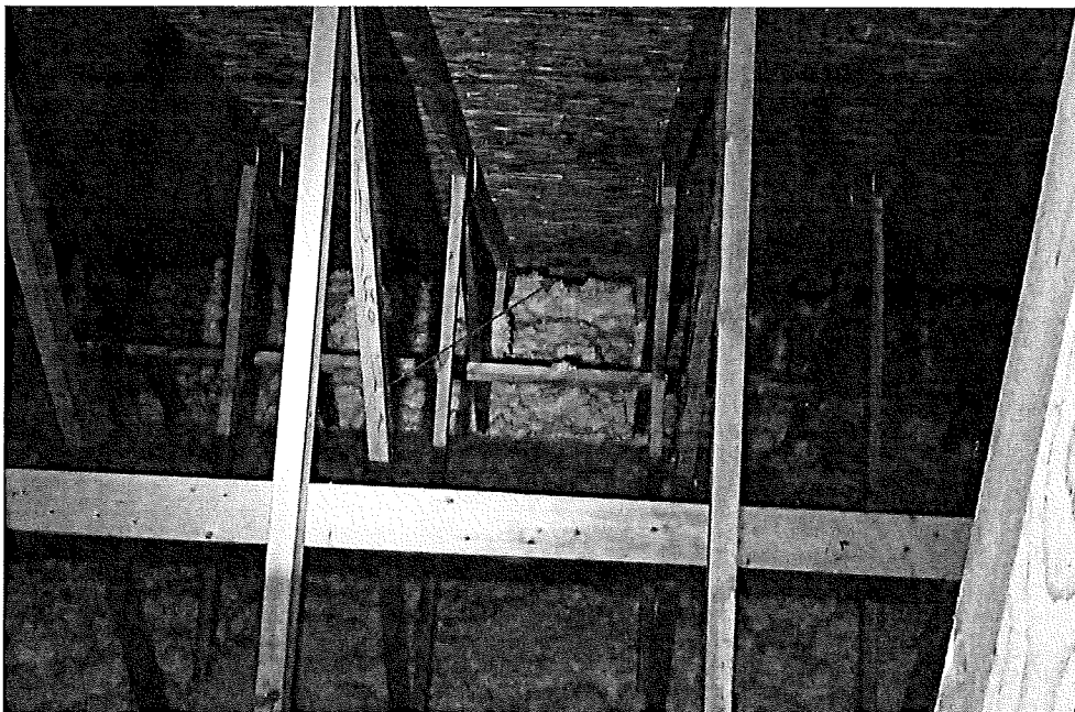
Photograph 14: Partial Air Chute
