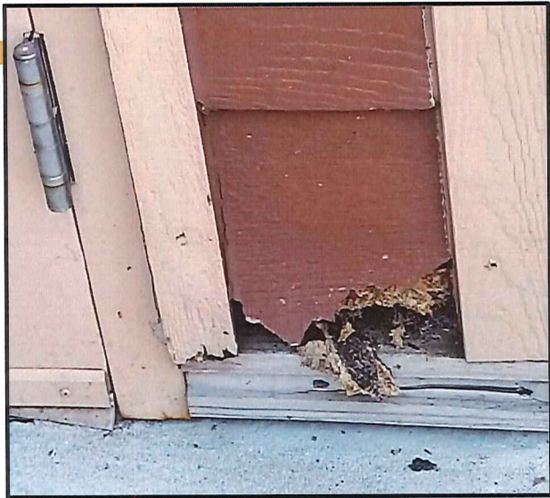
Masonite Siding Failing
