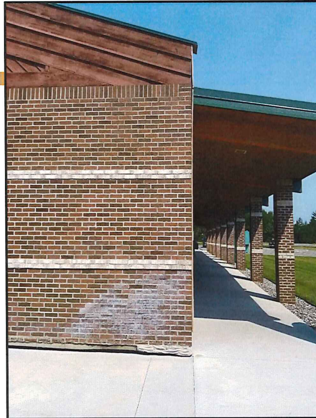
Efflorescence due to Water Penetration
