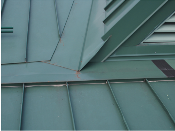
VALLEY FLASHING @ DORMER & ROOF SLOPE TRANSITION
