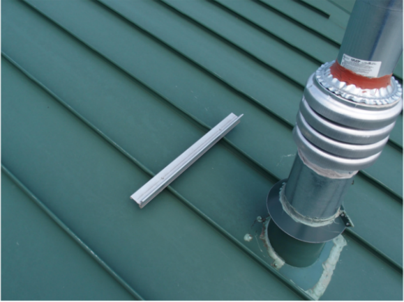
TYPICAL FLUE PENETRATION
