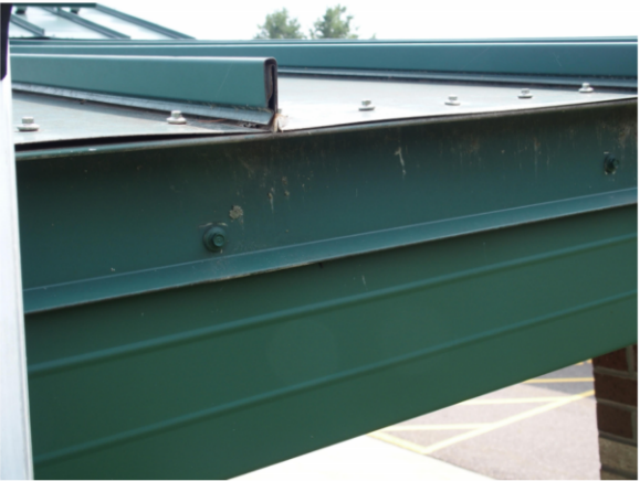
TYPICAL ROOF EDGE & STANDING SEAM
