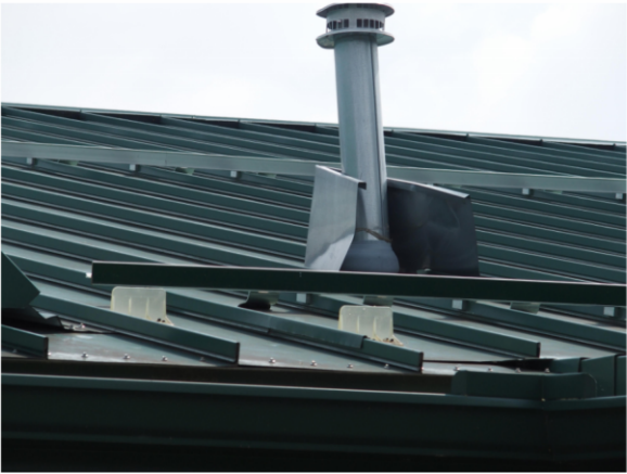
TYPICAL FLUE & ICE/SNOW STOP
